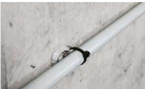
Flexible or rigid cable conduits with cable ties
