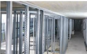
Drywall tracks to concrete and steel
