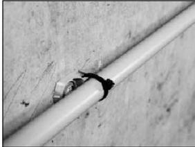
Flexible or rigid cable conduits with cable ties
