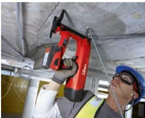
Threaded rod attachments to concrete
